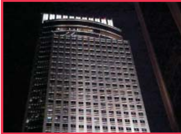
The First National Bank shines against the night sky, thanks to 384 metal halide fixtures mounted to the building's exterior.
