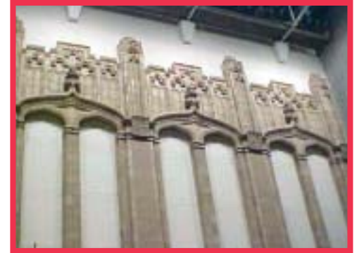
Some of the original architectural elements from the old Medical Arts Building have found new life in the tower's interior.
