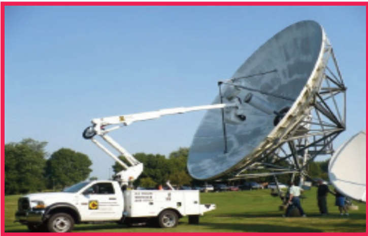
Troy Shannon performs general maintenance on an IPTV satellite
