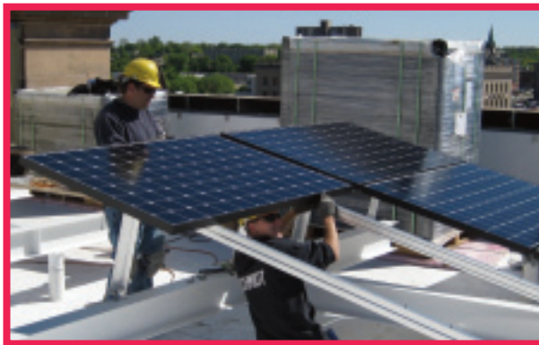
Workmen install solar panels at World Food Prize facility in Des Moines, IA
